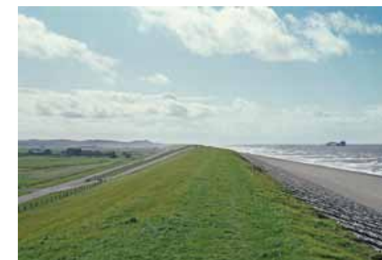
Bron: Van Oord Dredging and Marine Contractors
